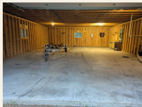
Inside the detached boat garage
